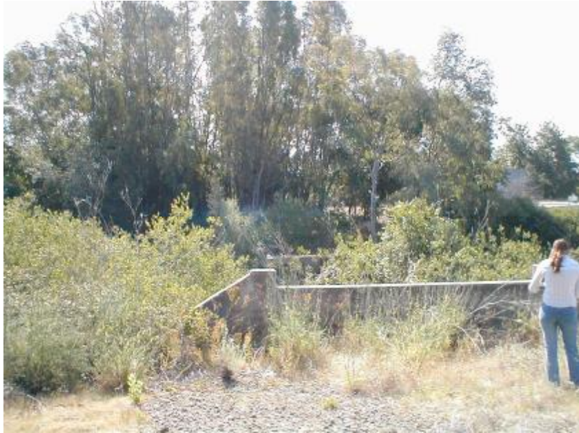
Taken at abandoned railroad crossing, approximately 1000 feet upstream of confluence with Butte Creek.
